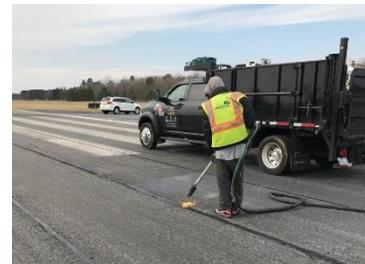
The Safety Preservation Airfield Maintenance (SPAM) program combines small preventative maintenance projects, such as pavement crack sealing and repainting runways, into a single statewide contract. This creates economies of scale and efficient, centralized administration of projects previously bid and managed as individual projects by local governments. And because the projects promote safety, DoA can fund them entirely, providing a cost savings to the airports.
